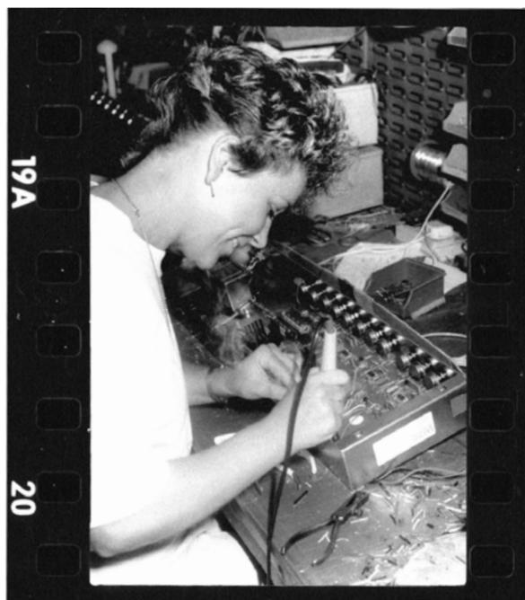
In the **Electronics department**, some amps are wired by hand using traditional 1962 construction methods, while others feature printed-circuit-boards automatically populated with up to six components per second. The boards are put into the chassis, wired-up and tested. At this point the panels, switches, transformers, and valve bases are also added manually.
